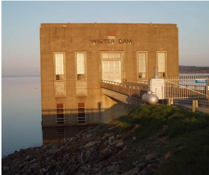
Figure 3: Lake Wister Dam
